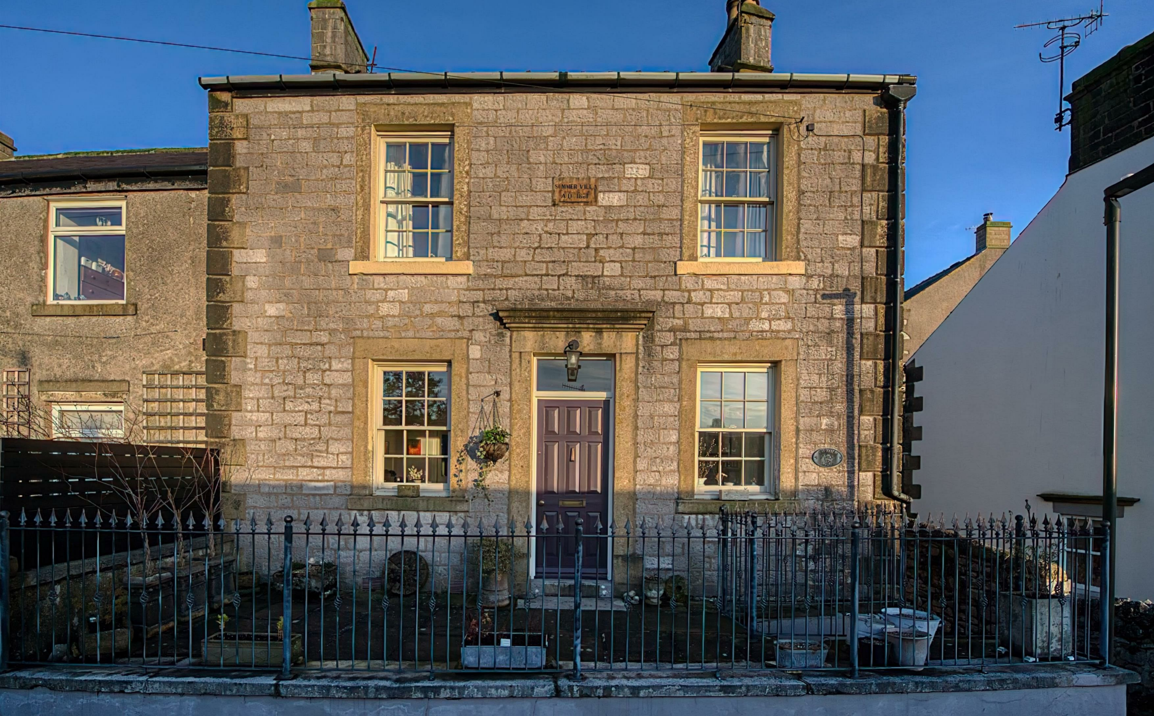
Summer Villa, Higher Terrace Road, Tideswell, Derbyshire, SK17 8NB
